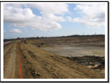
In addition to construction of the brine pond, G.R. Birdwell constructed plant roads, installed welded HDPE pipe for supply and return of brine, constructed concrete pads for various equipment foundations and piping to supply propane to the flare stack. At completion, over 30 acres were re-seeded.
